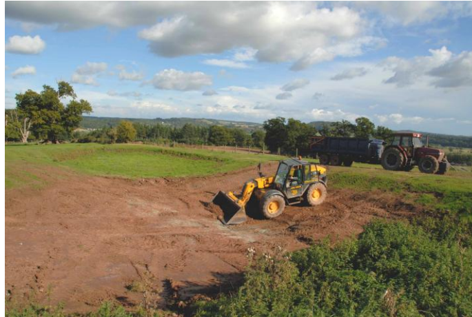
Digging out the old pond
